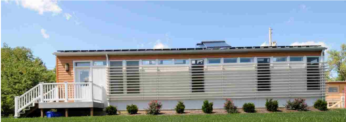
Figure 1.3. A View of the 2009 Solar House and Its Full Façade Louver Array
